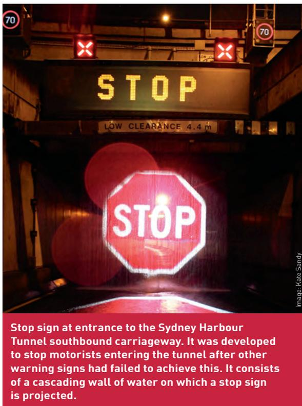
**Stop sign at entrance to the Sydney Harbour Tunnel southbound carriageway. It was developed to stop motorists entering the tunnel after other warning signs had failed to achieve this. It consists of a cascading wall of water on which a stop sign is projected.**
